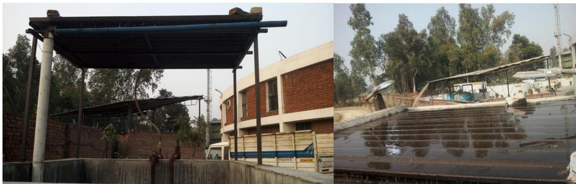
Fig 1 Showing 8 KL slope tank at leather industry
